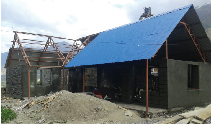
Construction is now complete!
