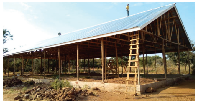
The newly constructed lunch pavilion
