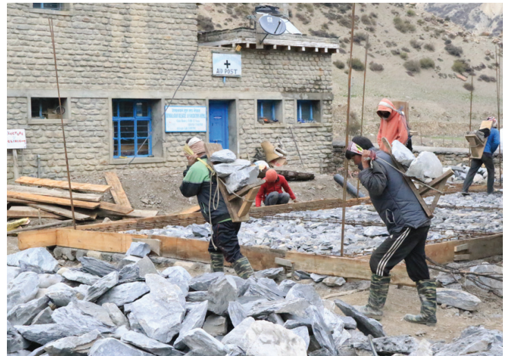
Medical Clinic construction in Nepal
