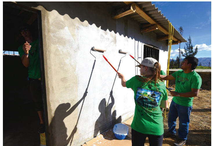
Volunteers painting the new computer center in Pashpa, Peru
