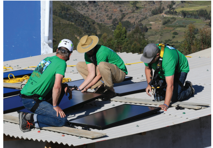
Installing solar panels
